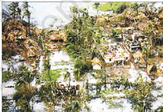
Destruction caused by a cyclone
