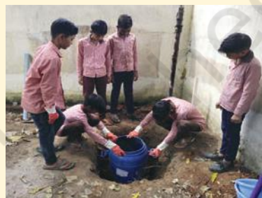
Figure 6.8: Students making a soakpit
