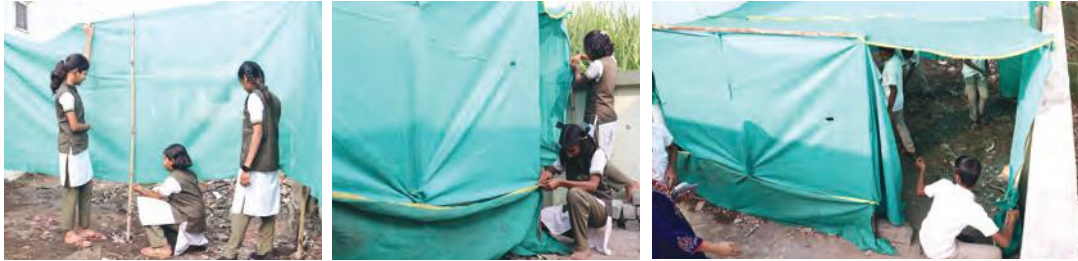
Figure 1.10: Installing the green shade-net
